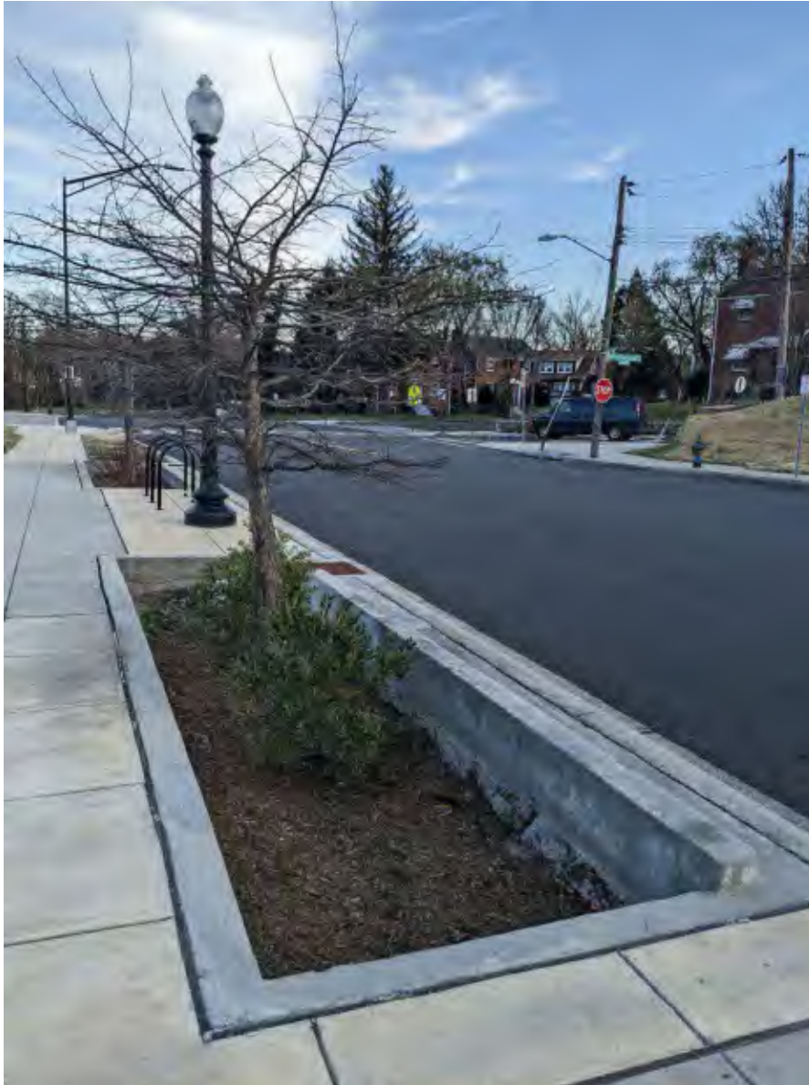
A street-side bioretention planter in Washington, DC.
