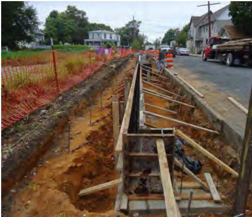
Bioretention under construction in Camden, NJ.
