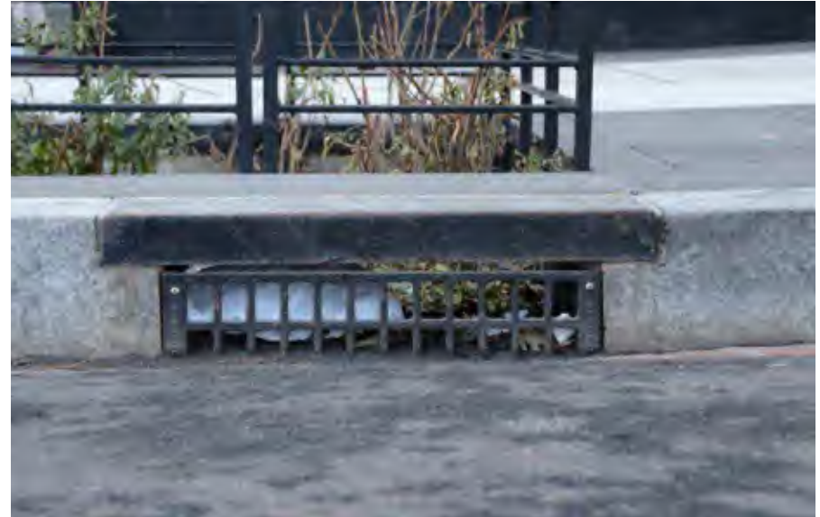
Debris clogs a grate leading into a bioretention facility.
