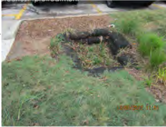
A vegetated bag forebay in Omaha, NE.
