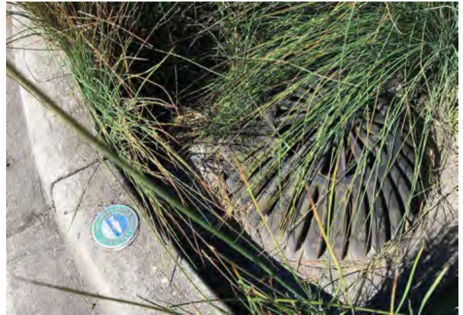
Vegetation overgrowth is blocking an overflow structure.
