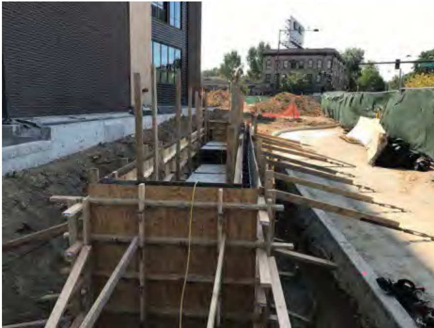
Bioretention under construction in Denver, CO.
