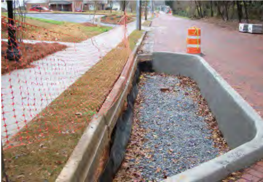
Bioretention under construction in Atlanta, GA.
