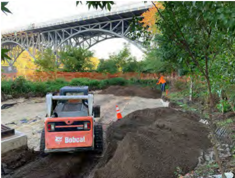
Soilless Soil Initiative project site during construction.
