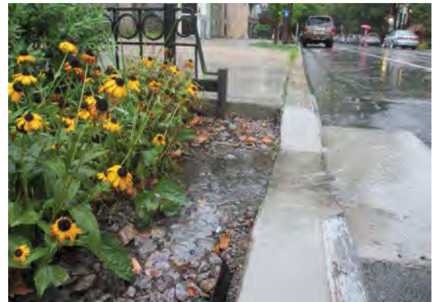
A well-designed inlet.
