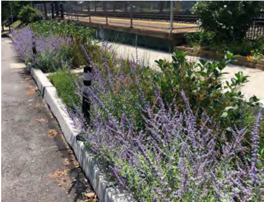
Stormwater curb extension bioretention in Philadelphia, PA.
