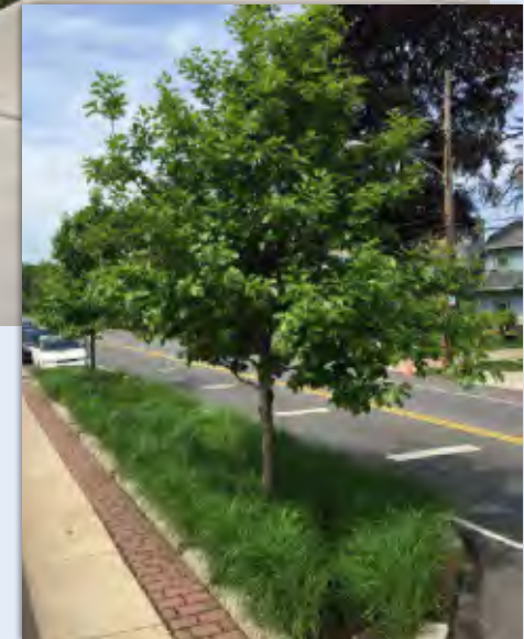
Bioretention facility with trees in Philadelphia, PA.
