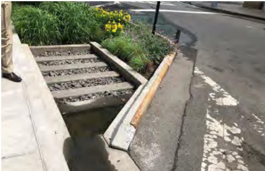
Concrete forebay in New York City, NY.
