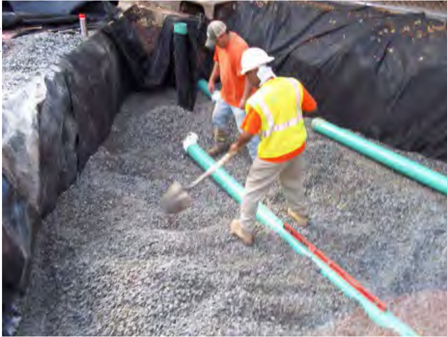
Installing aggregate media in Atlanta, GA.
