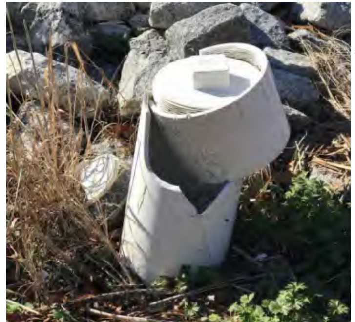
A broken cleanout.
