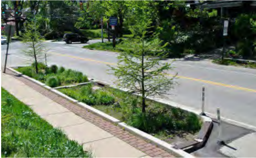
Stormwater curb extension in Philadelphia, PA.
