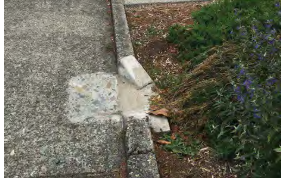
An angled curb cut in Seattle, WA.
