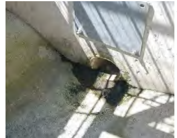
Underdrain outlet in an outlet box.
